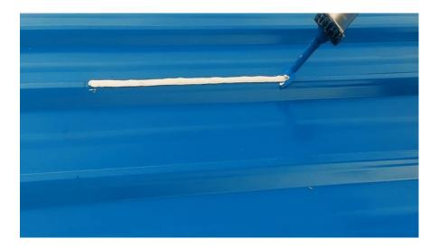
■ The glue length L2 is the same at the width of PV panel, distance between glue L1 should be less than 390mm, If module hanging part is above 50mm, use Aluminum support rail.
